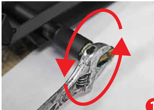
1 Removal of Natural Gas elbow and orifice
